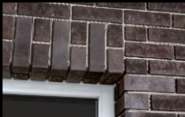
Window lintel perfectly replicated with angles.
