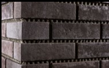
The finished surface. Grouting can be done after the appropriate drying time.
