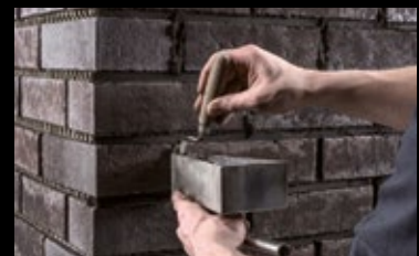
The vertical joints can be finished more easily with a smaller pointing trowel.
