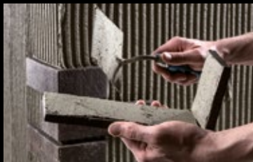
The corner angles are worked using the floating-buttering method.
