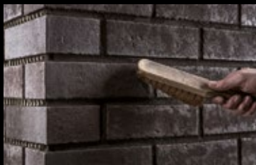
Sweeping out the joint gives it a corresponding structure.
