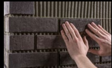
Use a string to plumb the clinker area. The clinker slips are pressed into the adhesive bed.
